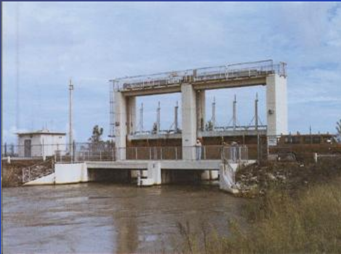
Typical flood / salinity control structure
