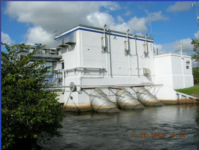
S-13 Pumping Station
